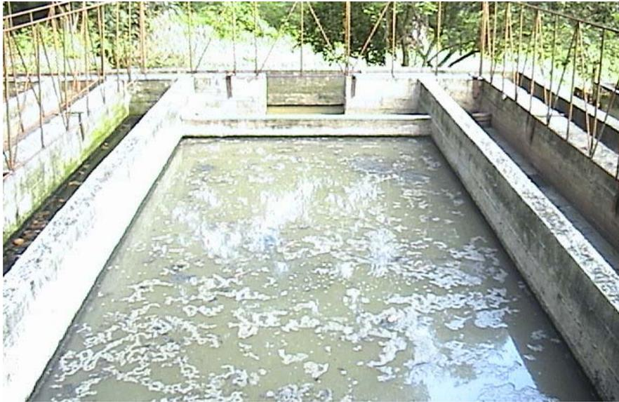
**Figura 2.2.** Tanque Imhoff.
