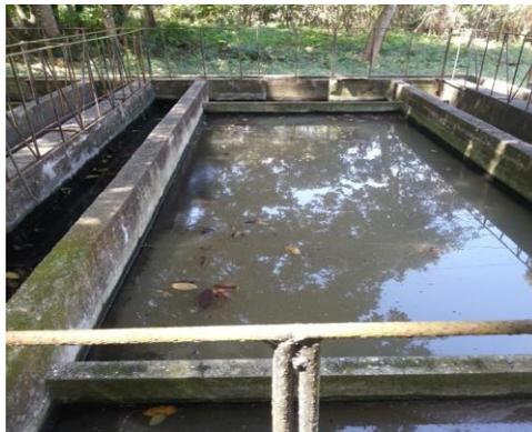
Figura 2.2 (Tanque Imhoff)
